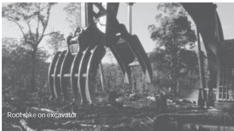
Root rake on excavator
