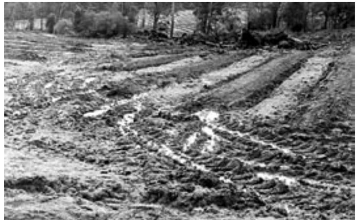
**Figure 2** is a job that started off well – cultivation stopped at the drainage depression. But the contractor who came in later to smooth the mounds must have been ill-advised. Working in wet weather he used the drainage depression as a turning area and, to use the vernacular, comprehensively “stuffed up” the careful work of his predecessor.
