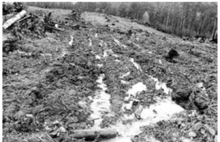
**Figure 4** shows the unfortunate effect of a culvert discharging over a shallow drainage depression in ex-native forest cultivated land. As the culvert was in position long before windrowing and cultivation occurred, topsoil loss and gullying could have been prevented by leaving the burnt area around the culvert exit undisturbed for about 50 m downslope.
