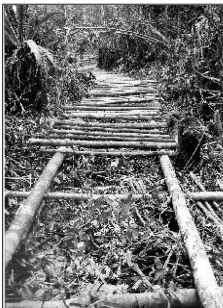
Kuda kuda track- interconnecting tracks are constructed by hand to every tree that is to be harvested.
